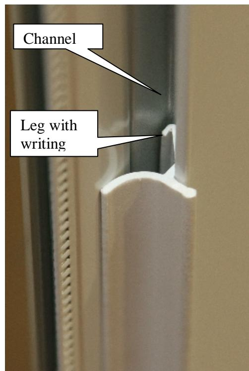
If the retainer or insert is loose the retainer may not be installed correctly. Ensure the retainer leg (with the writing) is not wedged between the insert and the door frame. The Retainer and insert will eventually fall out. The leg must be inside the channel on the frame.
